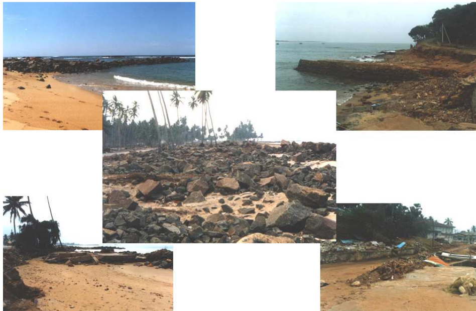
Plate 1: Disturbed revetments & groins in the Southern Coastal belt of Sri Lanka during tsunami
