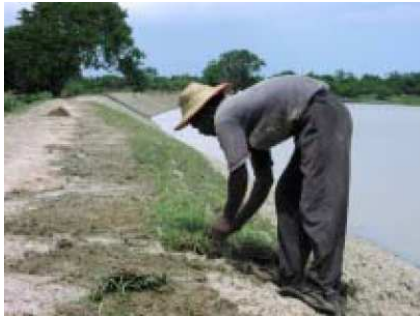
Turfing against erosion (5)
