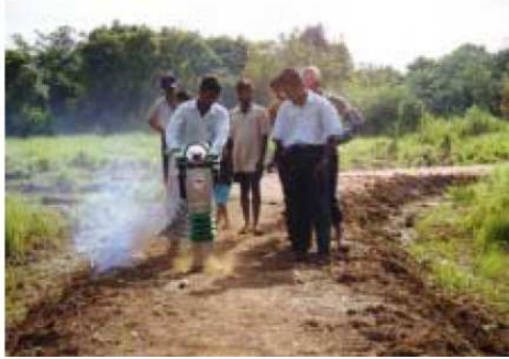
Compacting the bund (5)
